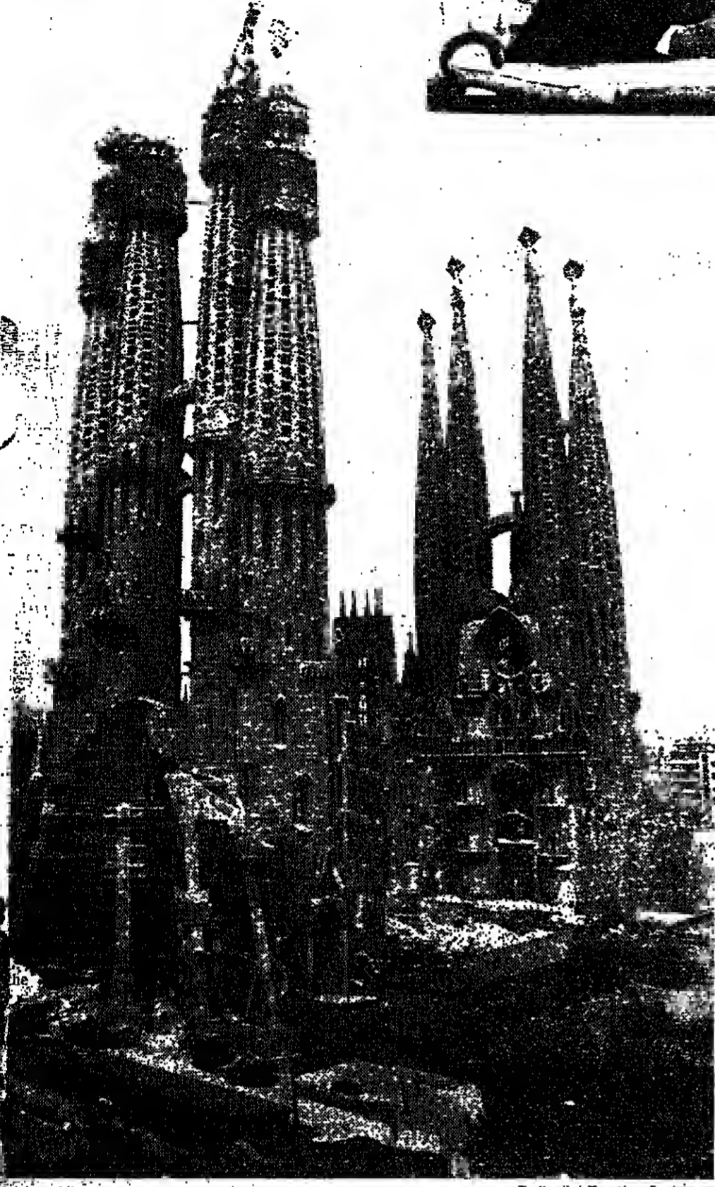
Joan Gaudí's Temple of the Holy Family in Barcelona, Spain. Above: Isidro Puig Boada, left, and Luis Bonet Garri, who are supervising the continued construction of the church.
